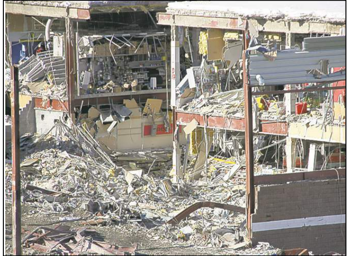
Figure 3-13 (Right): Collapsed Structure Elliot Lake, Ontario, 2012
